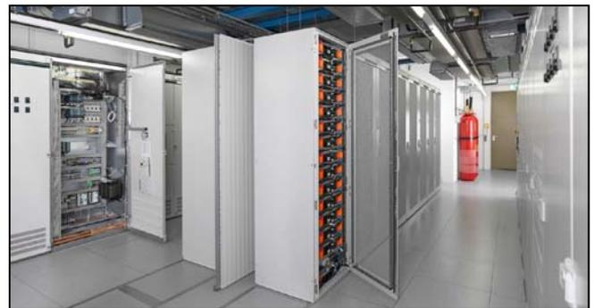
Figure 3: Battery energy storage system (BESS), Photo Siemens
