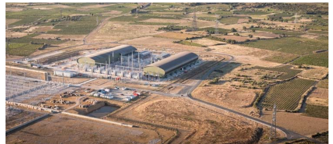
Figure 6. Inelfe Project, France-Spain, 2 x 1000 MW
